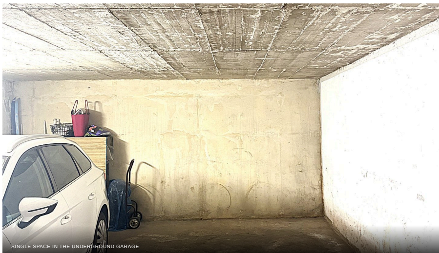
SINGLE SPACE IN THE UNDERGROUND GARAGE
